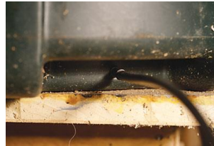
Fig 3. Connector with drainage tube inserted into bin
