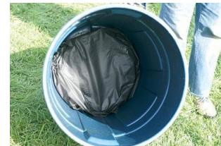
Fig 6. Cover drain pan with landscape fabric and install in bin
