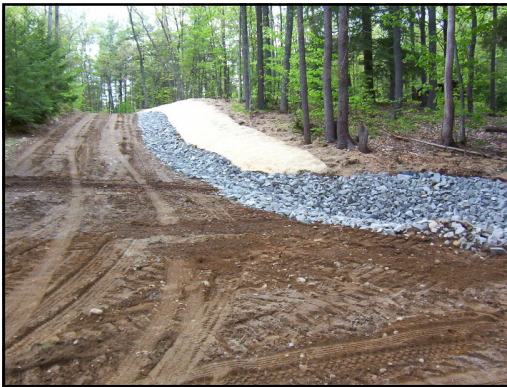
Camp road undergoing reconstruction. Road has been regraded to direct runoff to rip rap drainage ditch / detention structure along road side and new grass strip has been installed for soil stabilization.
